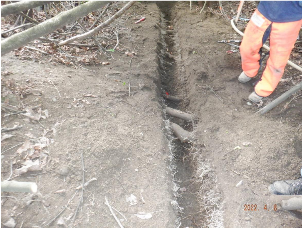
Air-excavated trench
